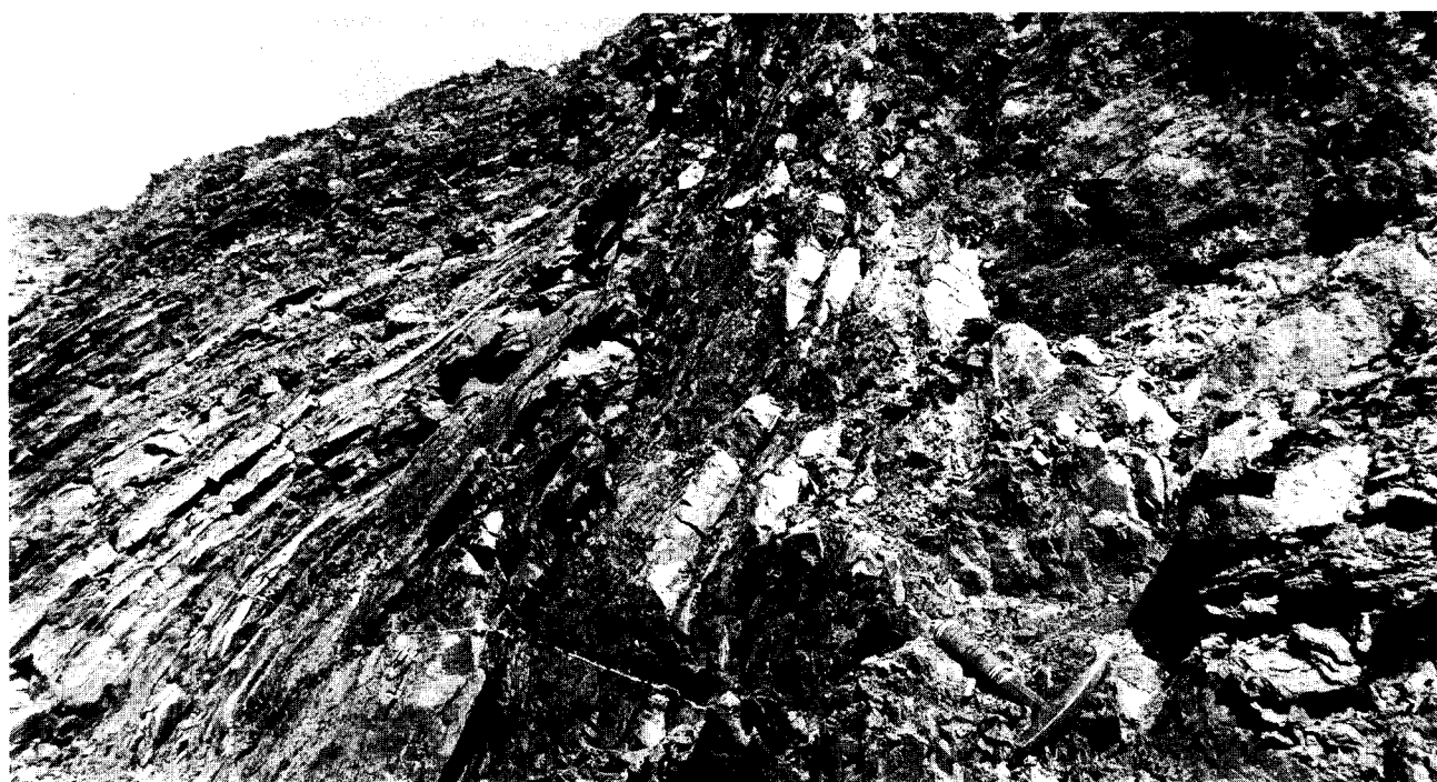
Fig. 5. Thin bedded parallel sequence of light- and dark coloured beds indicates rapid changes in the filling. The thickness of turbidites reached 3 - 7 cm. Tectonic contact of the filling with Wetterstein limestones can be seen in the right limb of the syncline. Photo by R. Marschalko.
